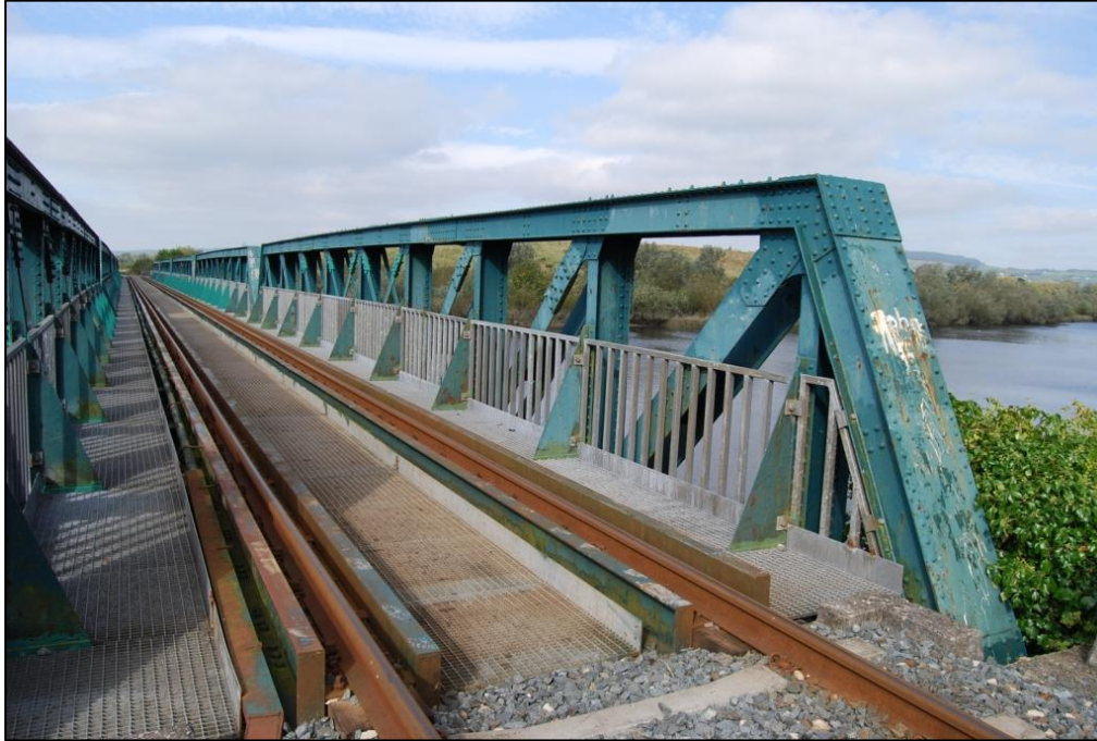
Photo 1. General view of Shannon River Bridge UBE16 in Limerick.
