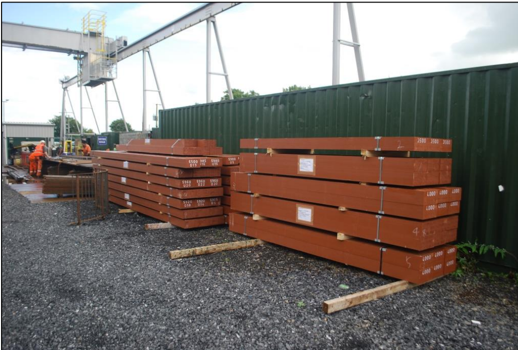
Photo 4. The FFU waybeams were manufactured in Japan by Sekisui Chemical Company Ltd and delivered to the Iarnród Éireann depot in Mullingar during August.
